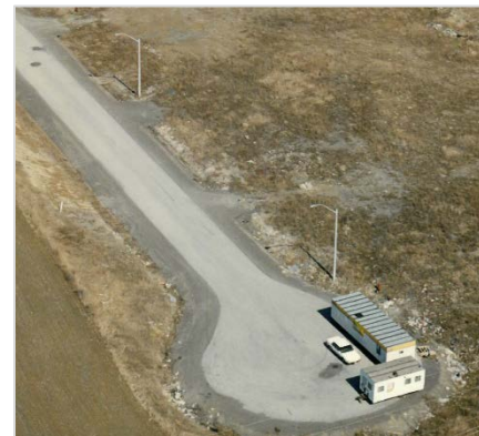
Photos from the 1996 shelter build
